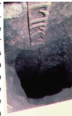
Areas of a mine that were once quite safe become dangerous after years of neglect. Decomposed rock often surrounds the top of a mine shaft and supporting timbers are frequently rotten. The entire area near an opening is often unstable and may cave into the shaft at any time, carrying an unwary trespasser with it.
